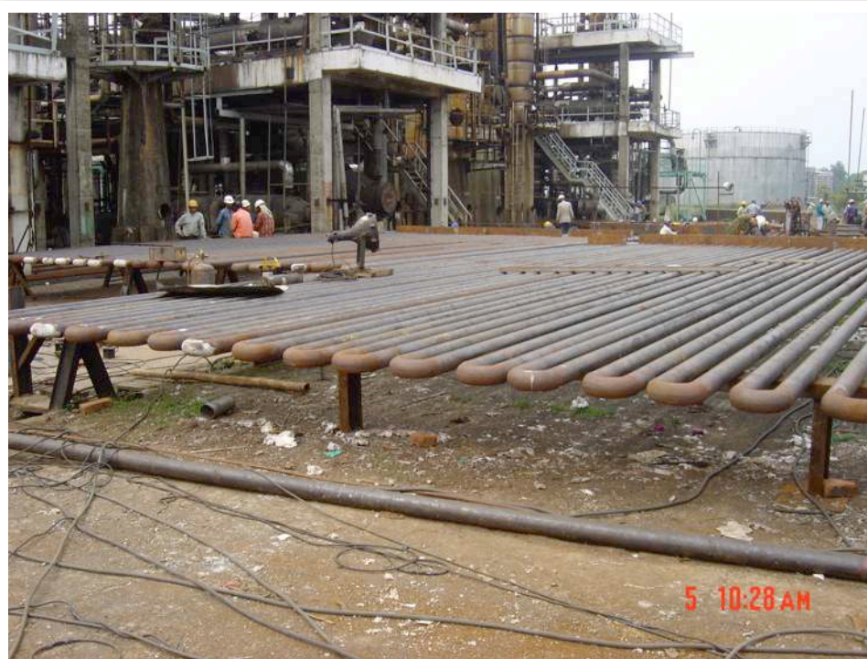
Pre-fabrication of Radiant Coils
