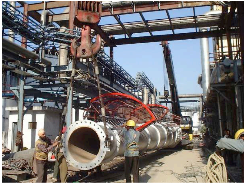
Stack fabricated in two modules complete with platforms and ladders
