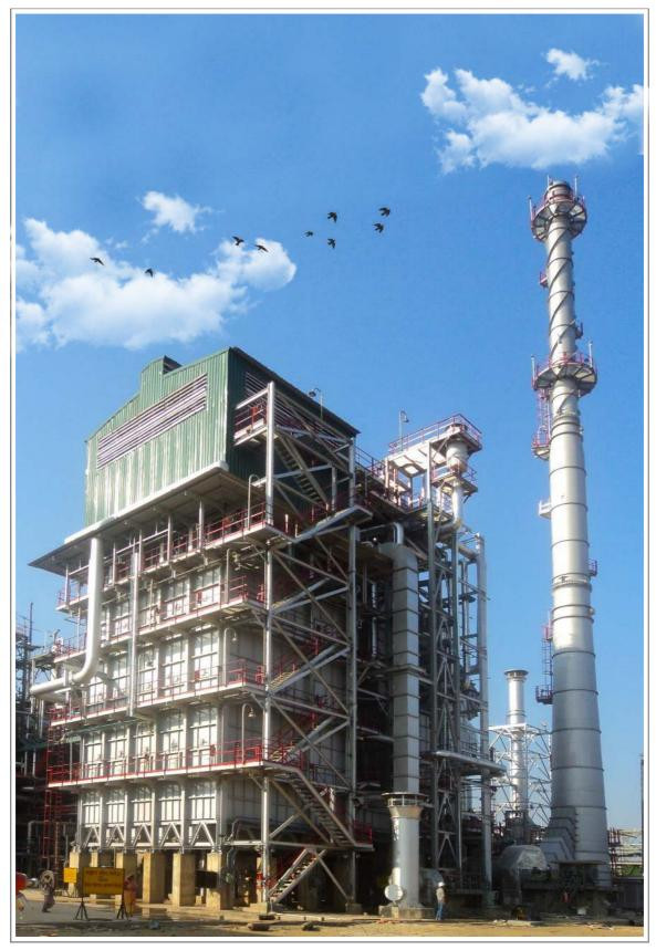
Steam Methane Reformer for HGU Unit (40.1 MMKcal/hr) fabricated and erected by Esteem Projects
