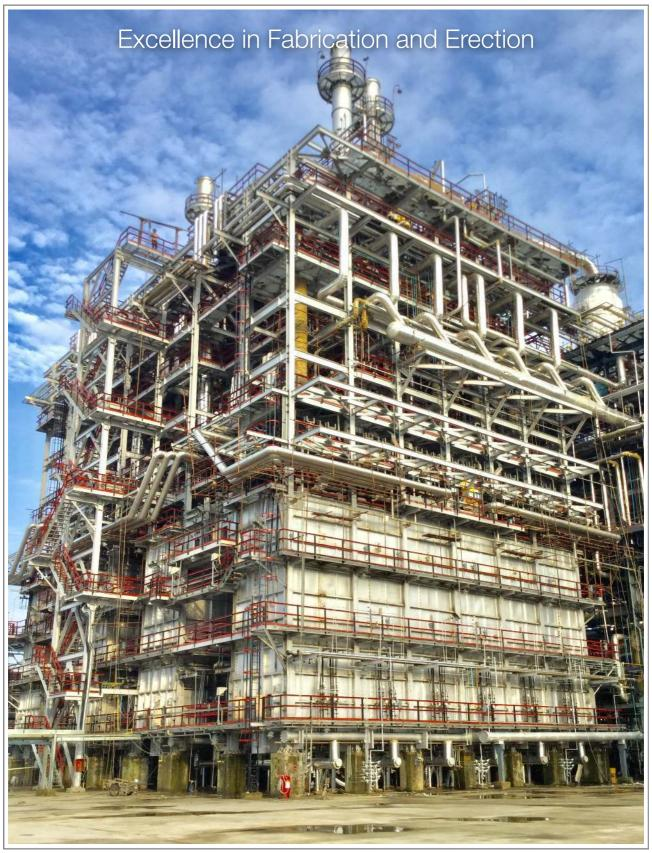
Naphtha Cracking Furnaces (39 MMKcal/hr x 4 Nos.) fabricated and erected by Esteem Projects
