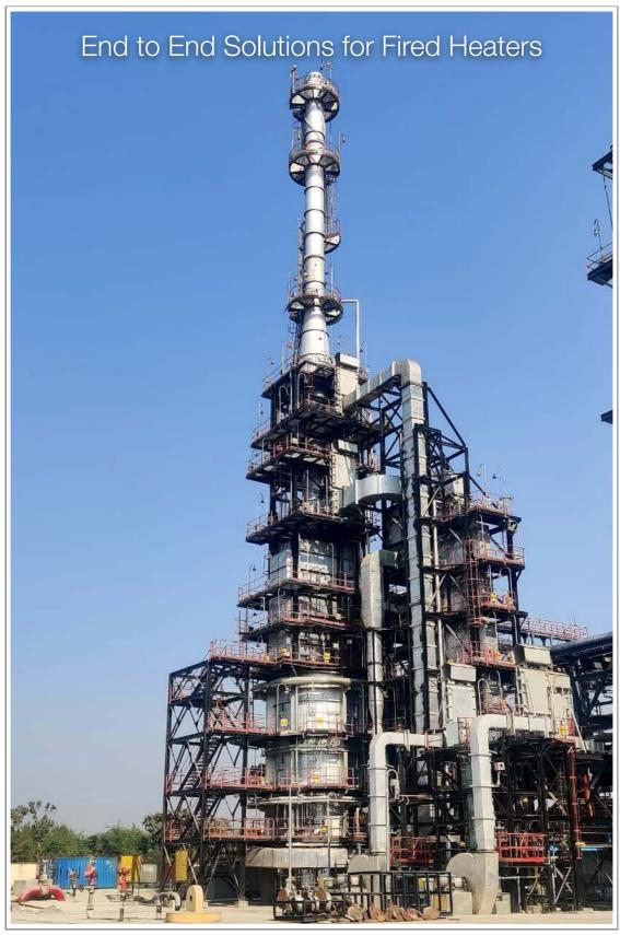
DHDT Unit Heater (5.26 MMKcal/hr) fabricated and erected by Esteem Projects
