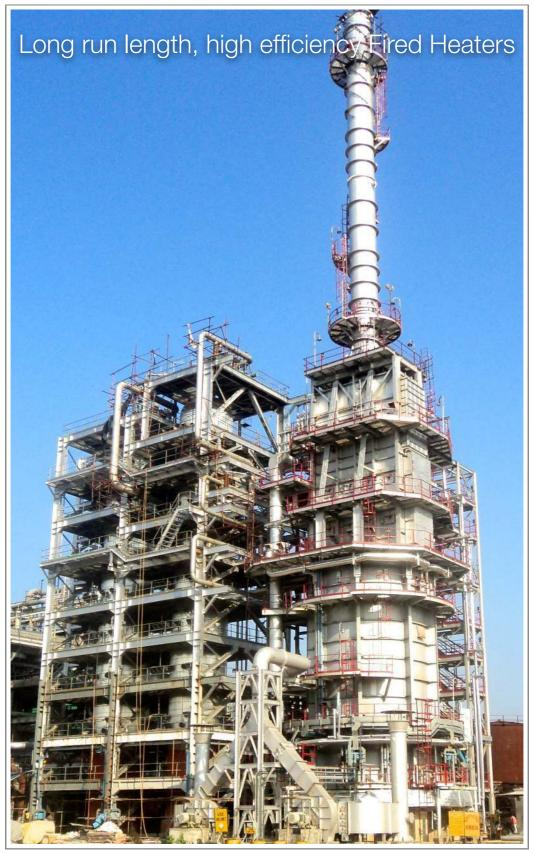
DHDT Unit Heater (12.7 MMKcal/hr) fabricated and erected by Esteem Projects
